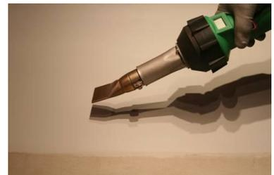
5. Weld the new (top) membrane to the dry and clean existing (bottom) membrane as per the usual procedure.
