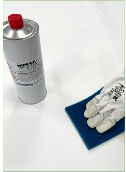
1. Remove all traces of dust, dirt, and deposits from the membrane.
