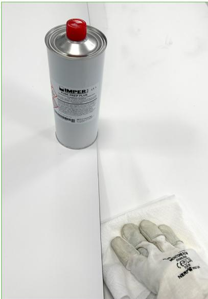
3. Clean with blotting paper and **FUSE PREP PLUS** cleaner until the surface and the paper appear clean.
