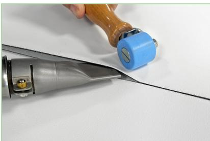
5. Weld the new membrane (top layer) onto the existing, clean, and dry membrane (bottom layer) using the manual welding technique.
